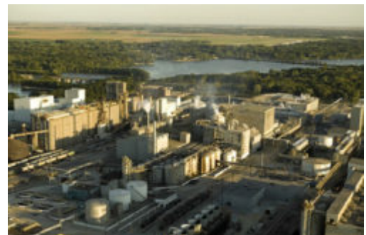
ADM's Agricultural Processing and Biofuels Plant, Decatur, IL. Credit: National Energy Technology Laboratory
