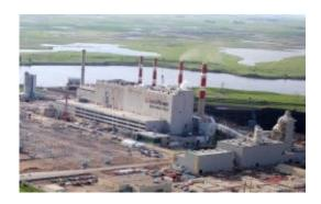
Unit 3 of the Boundary Dam Power Station in Estevan, Saskatchewan, has been converted for post-combustion CCS, producing over 1 million tonnes of CO2 per year – pipelined to oil fields in the south of the province to increase recovery. Photo: SaskPower vi
